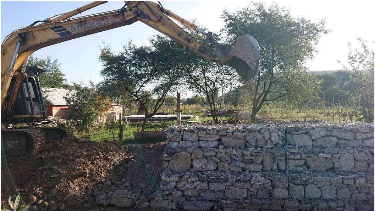
Protective gabion construction in the foothill village of Lanchyn, Nadvirna Raion. September 2020
